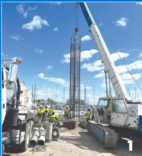
[1]: A crane is used to place steel reinforcement in the foundation for the overhead sign structures. [2]: Conduit is laid in protected trenches in many corridors throughout the project. [MAIN]: A new overhead sign structure is assembled in preparation for installation.
