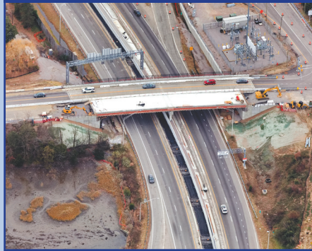
MALLORY STREET BRIDGE
