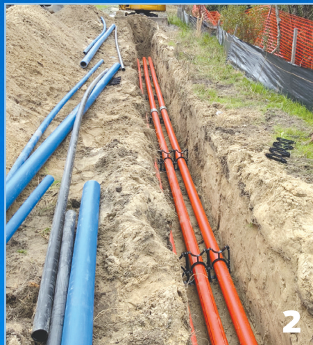
[1]: A crane is used to place steel reinforcement in the foundation for the overhead sign structures. [2]: Conduit is laid in protected trenches in many corridors throughout the project. [MAIN]: A new overhead sign structure is assembled in preparation for installation.
