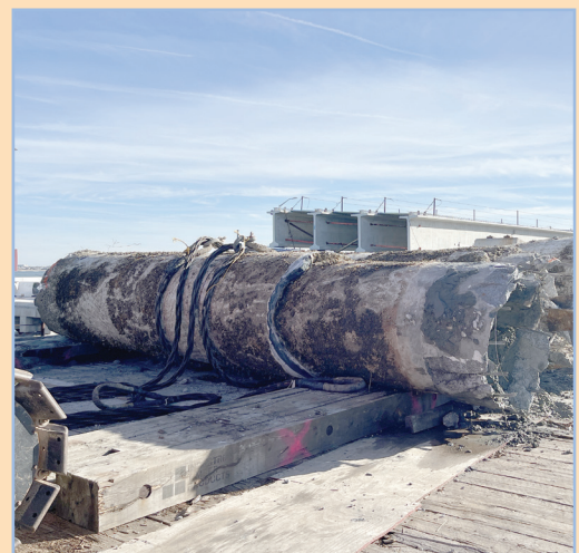
Support piles of the original bridge removed from the water.
