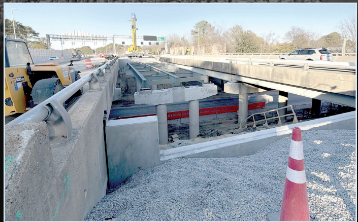
Crews place girders for the bridge over W. Bayview Boulevard.
