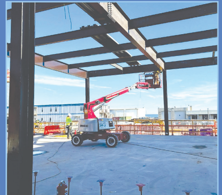
Steel beams provide structural support for the ventilation building on the South Island.
