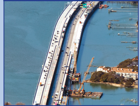
WILLOUGHBY BAY BRIDGE
