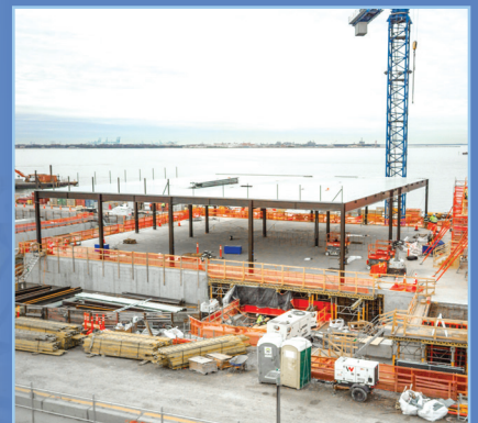
Progress of building construction on the South Island.
